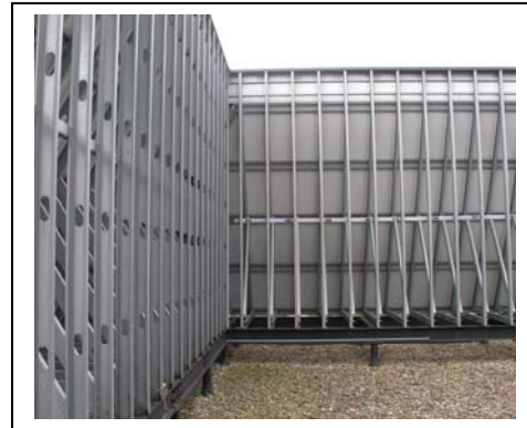
(Left) Roof Screen Wall Framing Detail (Above) Roof Screen Wall and roofing system
